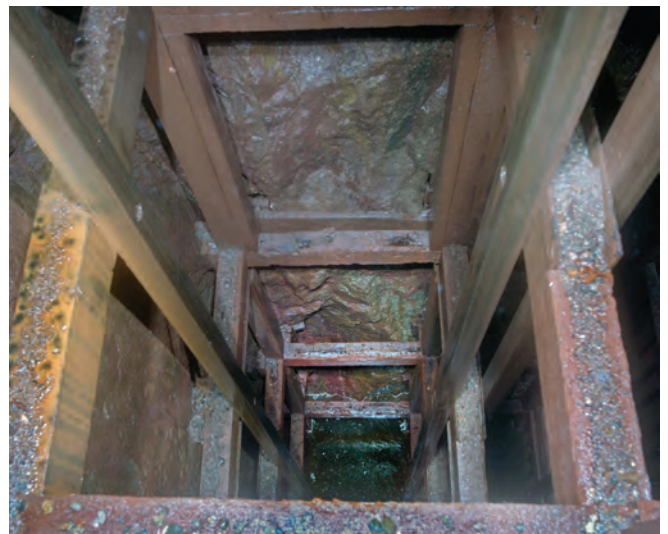
Looking down Victory Shaft from level 3 in 1995. The shaft is flooded up to the level of the drainage adit. The water level in the shaft remains the same today.
